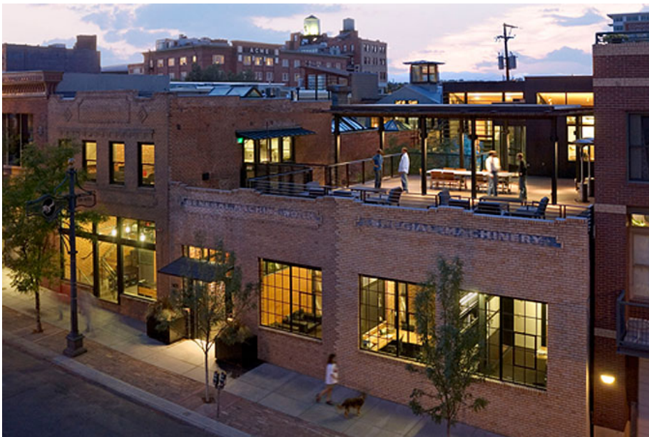
An adaptive re-use of a 1900s building. New building materials (windows and doors) are compatible with the historic materials.
