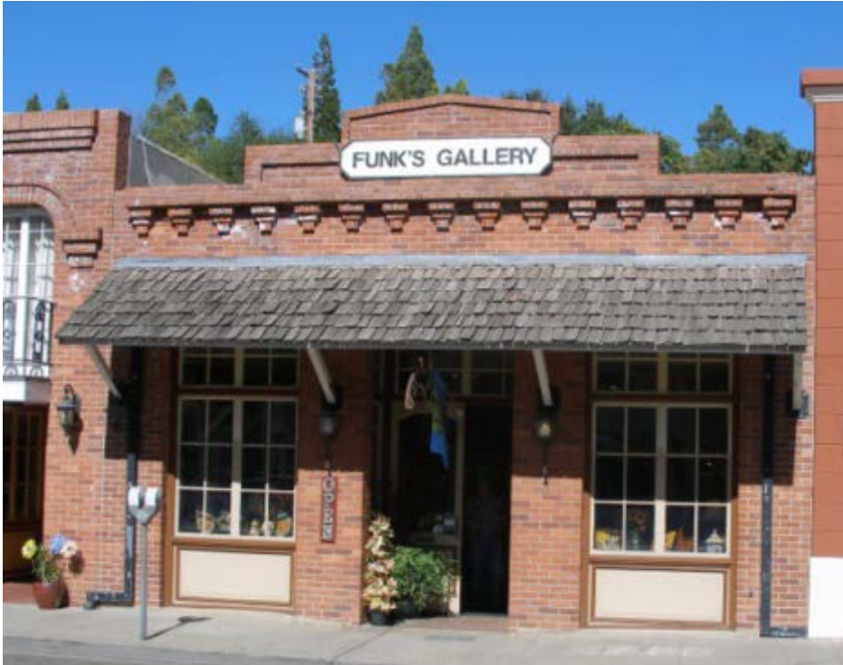
Use of recessed entry, framed windows, awning, clean roofline, and traditional building materials.
